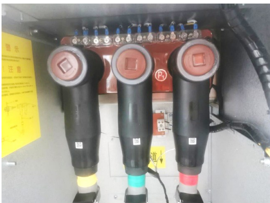
Ring main unit – before and after installing temperature-sensing insulating plugs
