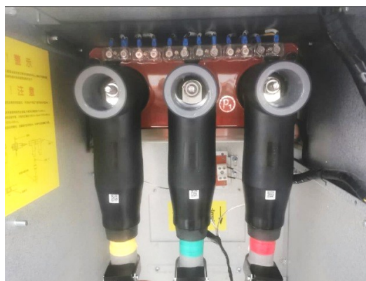
Ring main unit – before and after installing temperature-sensing insulating plugs
