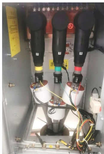
Ring main unit – after installing the temperature-sensing insulating plug and back cover
